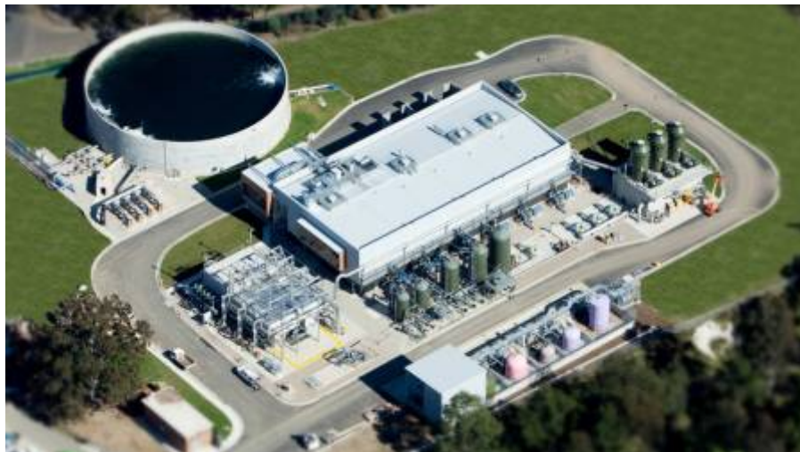
Figure 6: Sydney desalination plant [8]
